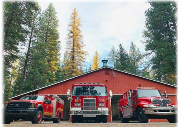
Station 704 in Camp Sherman got a big facelift with new paint, windows and updated signage.
