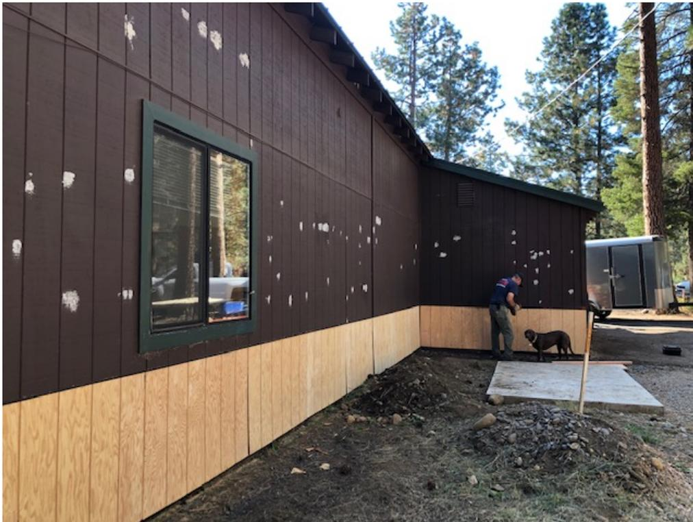
PICTURED ABOVE – STATION 704 REPAIRS IN 2022 INCLUDED REPLACEMENT OF DAMAGED SIDING, NEW EXTERIOR PAINT, IMPROVEMENTS TO THE FOYER, NEW CONCRETE SLAB AND DORM WINDOWS
